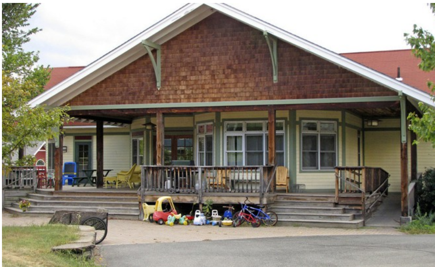
Figure 2: Porch around common house in one cohousing community.
